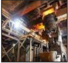
IRON & STEEL PLANT
